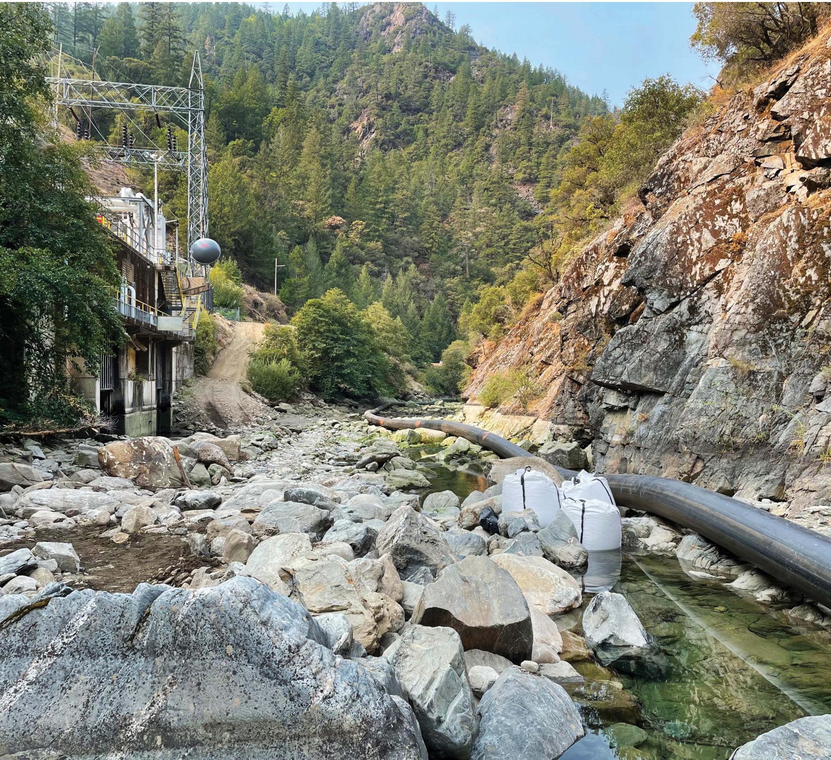
Middle Fork Interbay - Powerhouse Tailrace (Dewatered)
