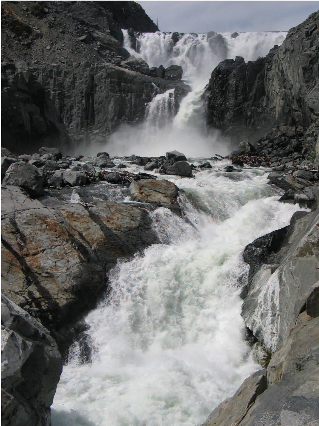
Hell Hole Reservoir Spillway
