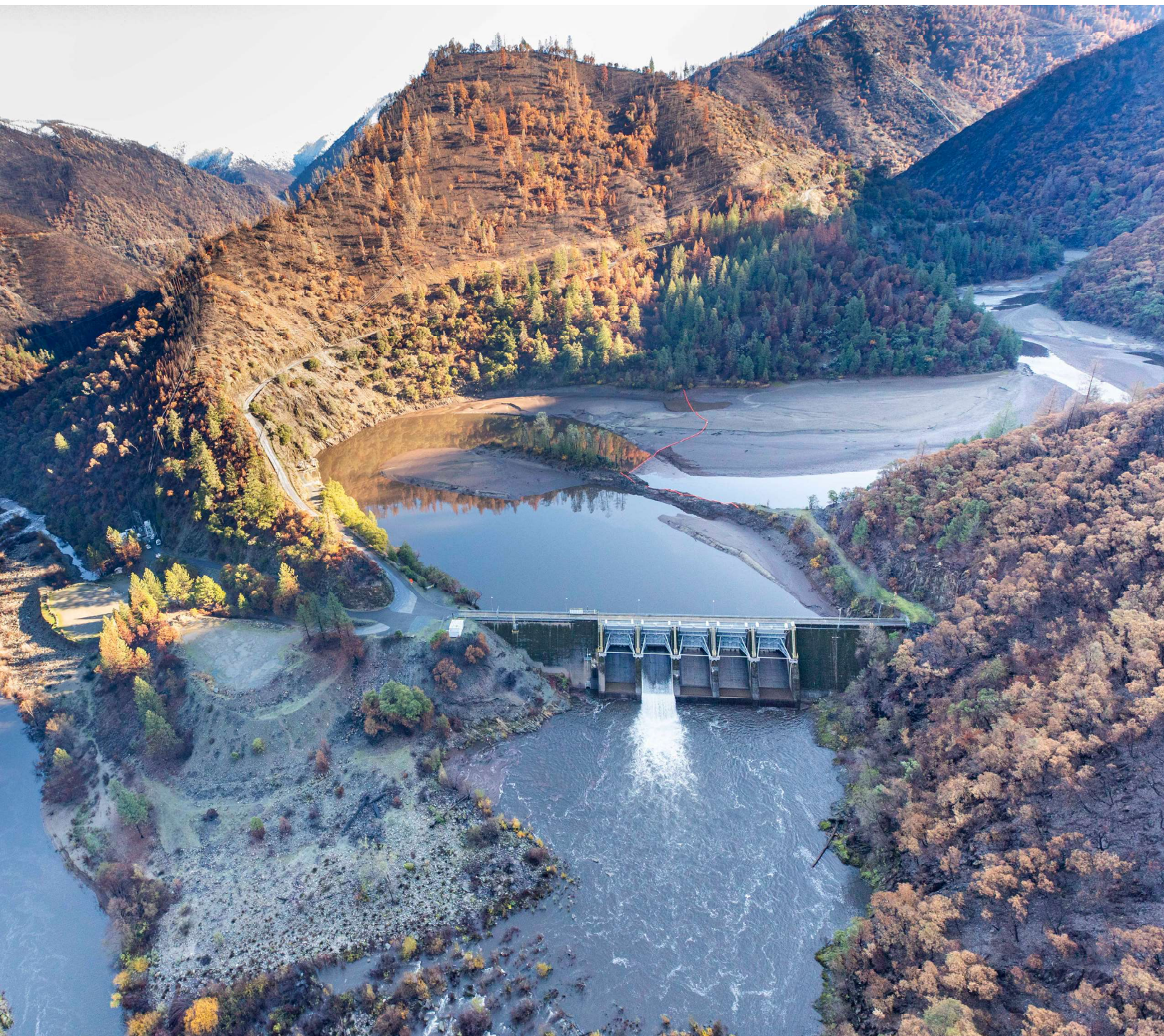
Ralston Afterbay Dam
